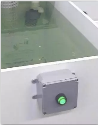
IN-USE ON A TANK
